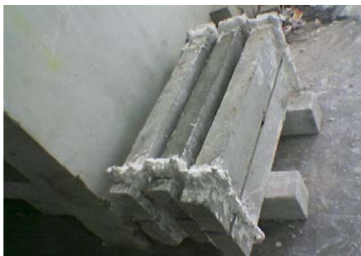
Figure (3): Beams before fire
