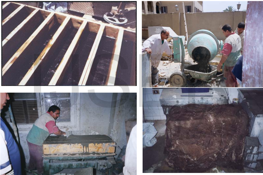
Figure (2): Preparing of beams
